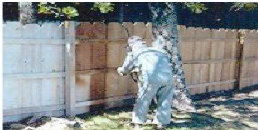
Applying TWP 100 Series Cedertone Natural to a cleaned, weathered cedar fence.
