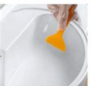
Smooth out the edges and flatten the material with the scraper.
