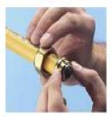
Step 3: Slide nut over retainer and hand tighten.
