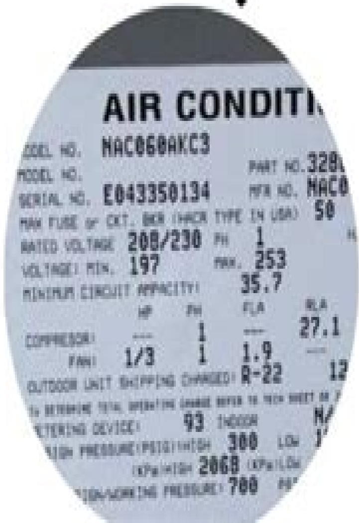
OUTDOOR UNIT (AIR CONDITIONER/HEAT PUMP)
